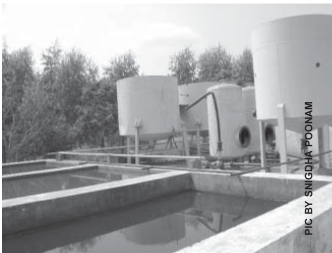
Pictures (clockwise): Electricity generation plant; Water recycling system and a worker cutting wood for feeding into the plant.
